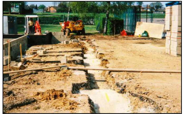
Digging the foundations for the amenities block
