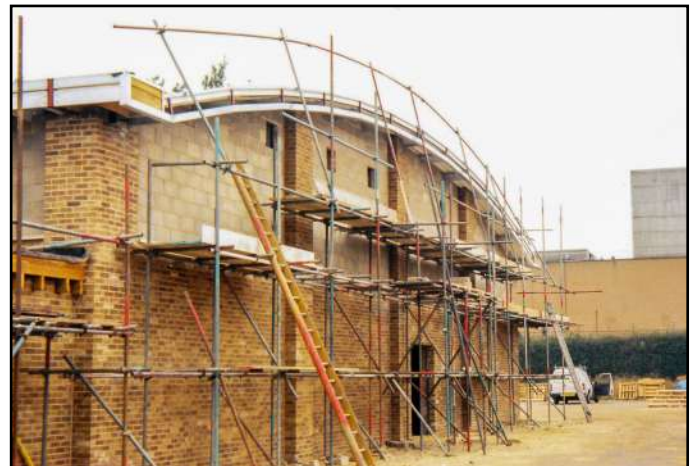
Now it's beginning to look like a building!
