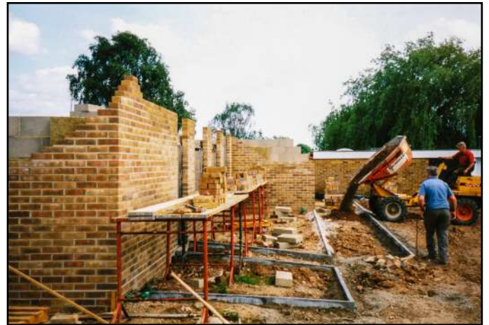
The walls of the amenities block start to rise
